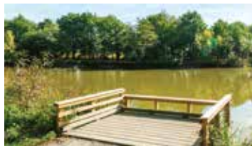
PONTON PMR, MONTBERT
